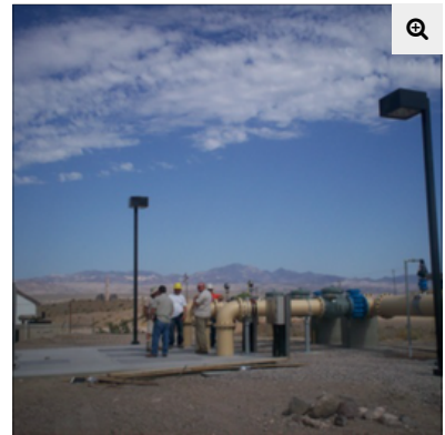
Lift Station Wet Well
