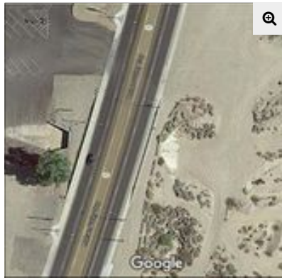
Secret Pass Culvert in Community Park
