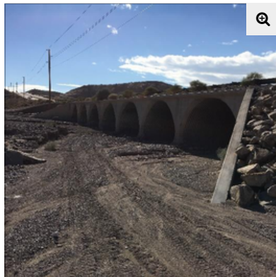
Grade Control Structure
