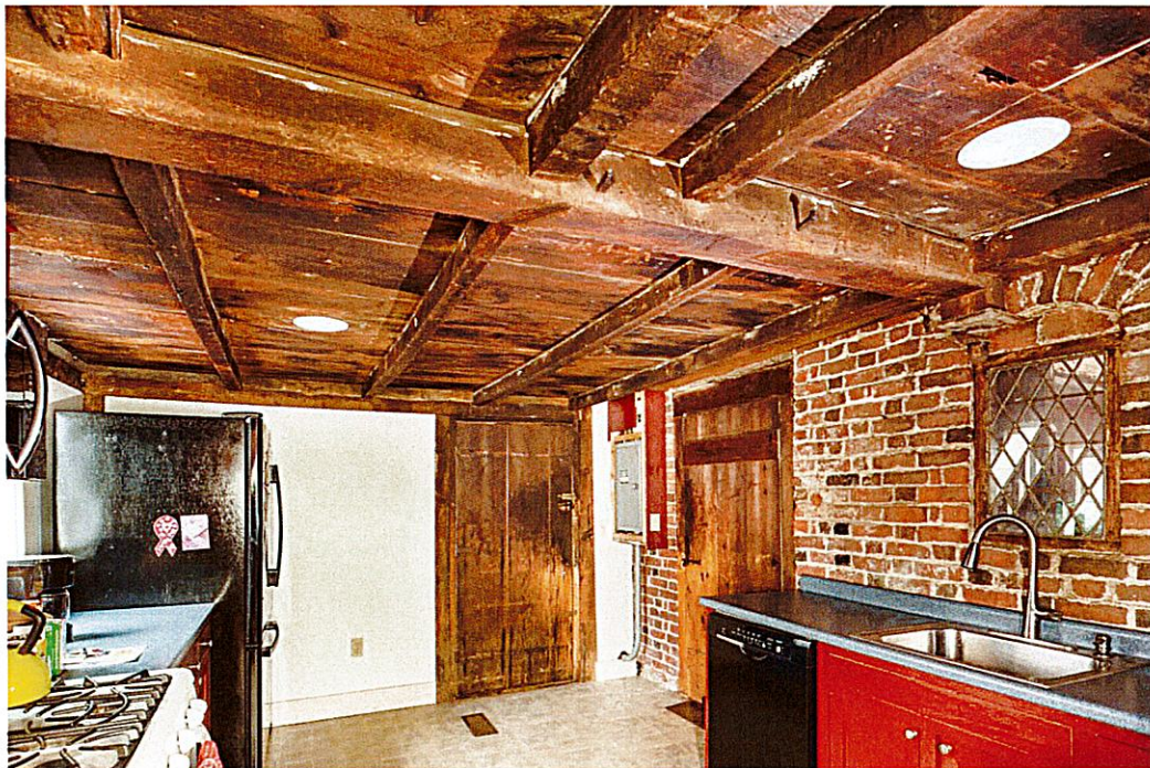
Exhibit B - MA: Haverhill, 790 East Broadway, PEASLEE GARRISON Lean-To, looking southwest (RSID #502299)
