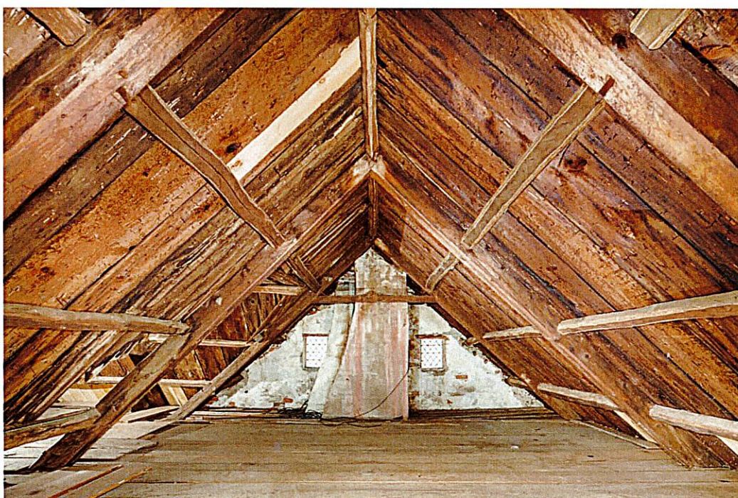
Exhibit B - MA: Haverhill, 790 East Broadway, PEASLEE GARRISON Main Block: Attic, looking east (RSID #502329)
