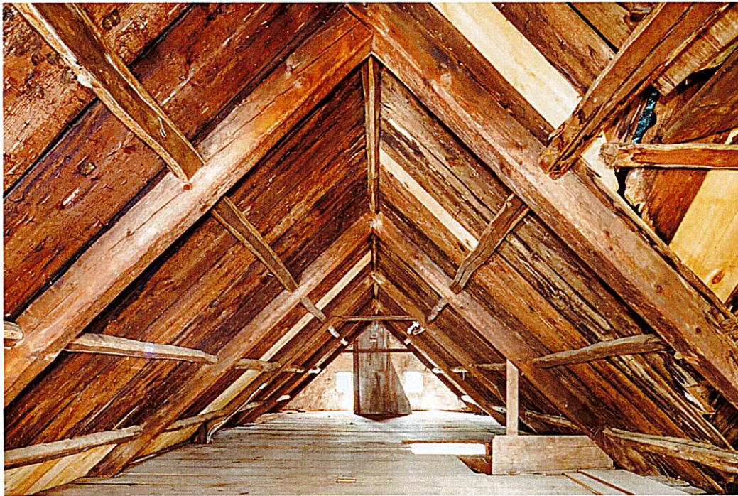
Exhibit B - MA: Haverhill, 790 East Broadway, PEASLEE GARRISON Main Block: Attic, looking west (RSID #502330)
