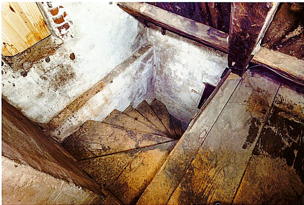
Exhibit B - MA: Haverhill, 790 East Broadway, PEASLEE GARRISON Rear Ell: Attic, looking northeast down the North Stair (RSID #502326)
