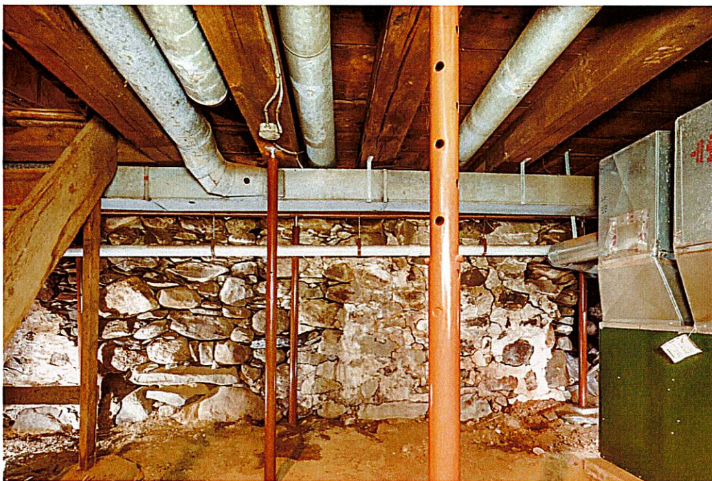
Exhibit B - MA: Haverhill, 790 East Broadway, PEASLEE GARRISON Main Block: Cellar, looking north (RSID #502338)
