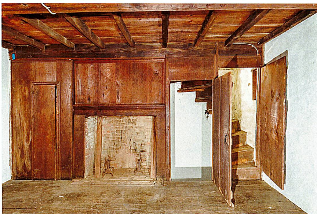
Exhibit B - MA: Haverhill, 790 East Broadway, PEASLEE GARRISON Rear Ell: Northeast Chamber, looking north (RSID #502321)
