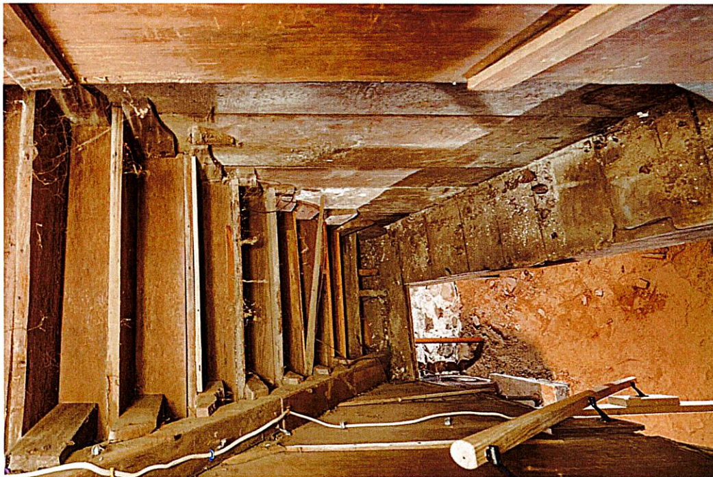
Exhibit B - MA: Haverhill, 790 East Broadway, PEASLEE GARRISON Main Block: Main Entry Hall, looking south (RSID #502287)
