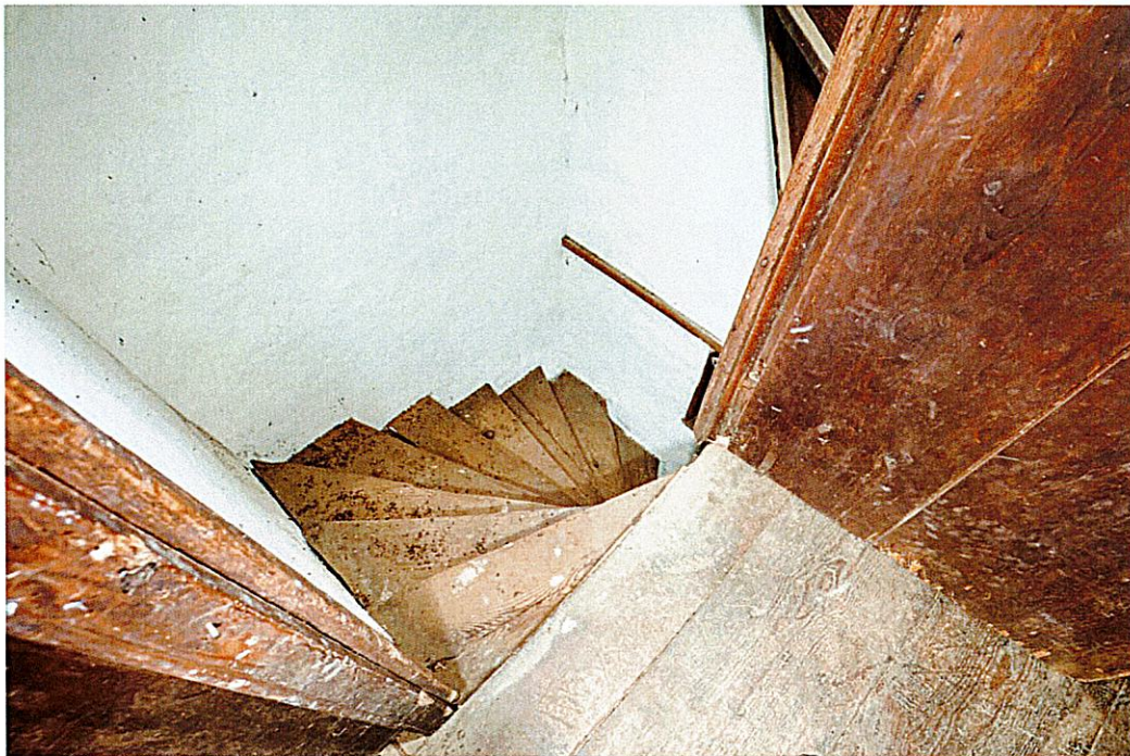
Exhibit B - MA: Haverhill, 790 East Broadway, PEASLEE GARRISON Rear Ell: North Stair, looking northeast (RSID #502323)
