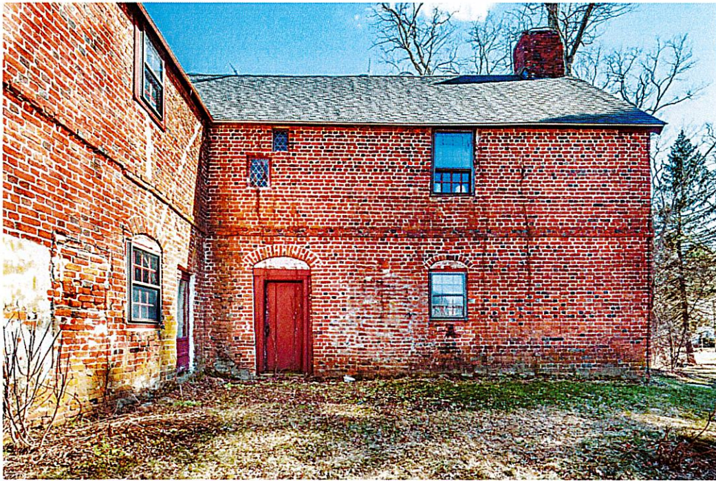
Exhibit B - MA: Haverhill, 790 East Broadway, PEASLEE GARRISON Main Block & Rear Ell: North & West Elevations (RSID #502280)
