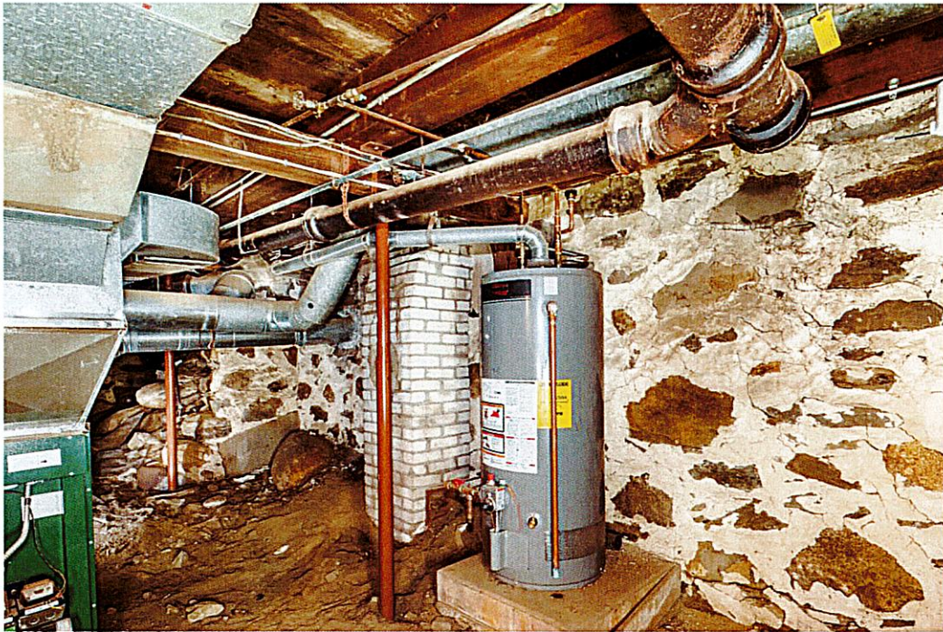
Exhibit B - MA: Haverhill, 790 East Broadway, PEASLEE GARRISON Main Block: Cellar, looking northeast (RSID #502335)
