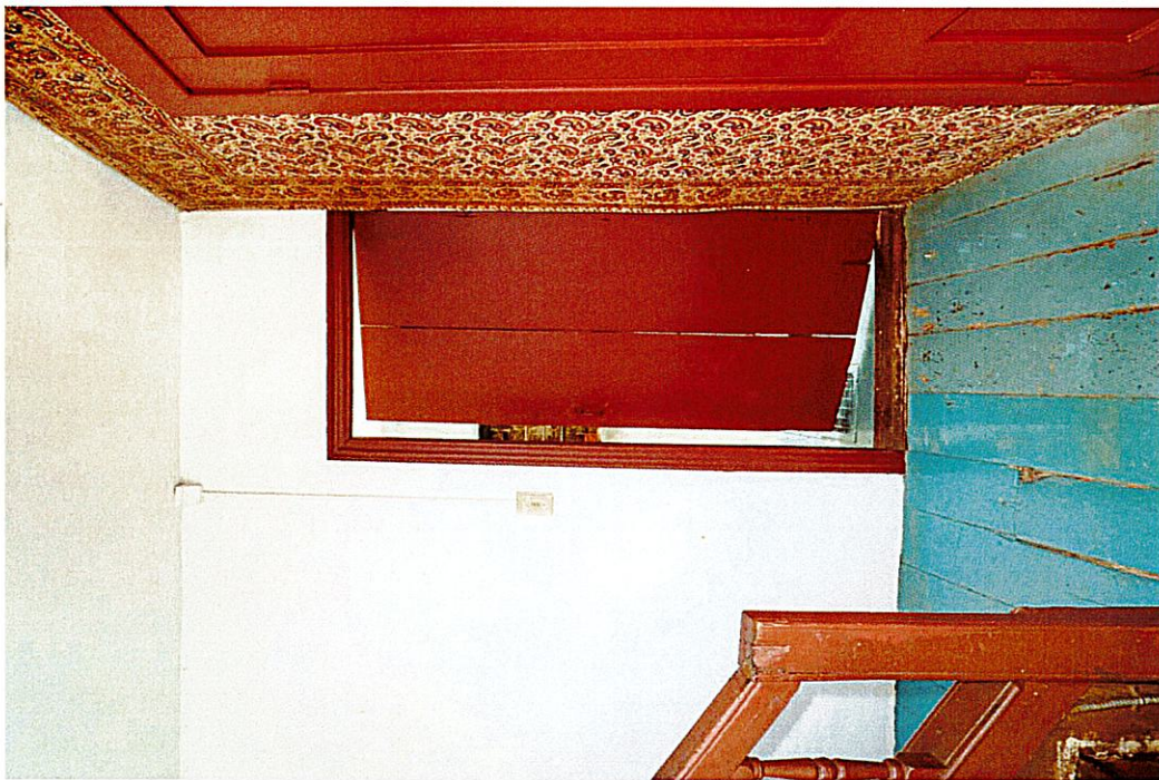
Exhibit B - MA: Haverhill, 790 East Broadway, PEASLEE GARRISON Main Block: Main Stairhall, looking east (RSID #502310)
