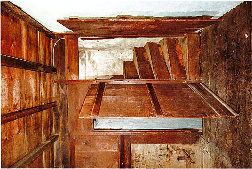
Exhibit B - MA: Haverhill, 790 East Broadway, PEASLEE GARRISON Rear Ell: Northeast Chamber, looking north (RSID #502322)
