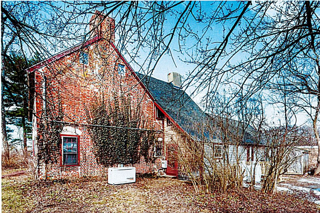
Exhibit B - MA: Haverhill, 790 East Broadway, PEASLEE GARRISON Main Block, Rear Ell, Lean-To, & North Addition: South & East Elevations (RSID #502274)
