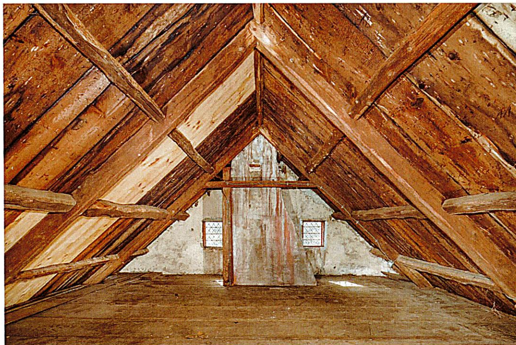
Exhibit B - MA: Haverhill, 790 East Broadway, PEASLEE GARRISON Main Block: Attic, looking west (RSID #502331)
