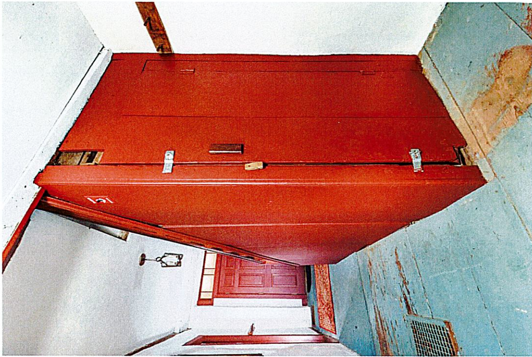
Exhibit B - MA: Haverhill, 790 East Broadway, PEASLEE GARRISON Main Block: Main Entry Hall, looking southwest (RSID #502286)
