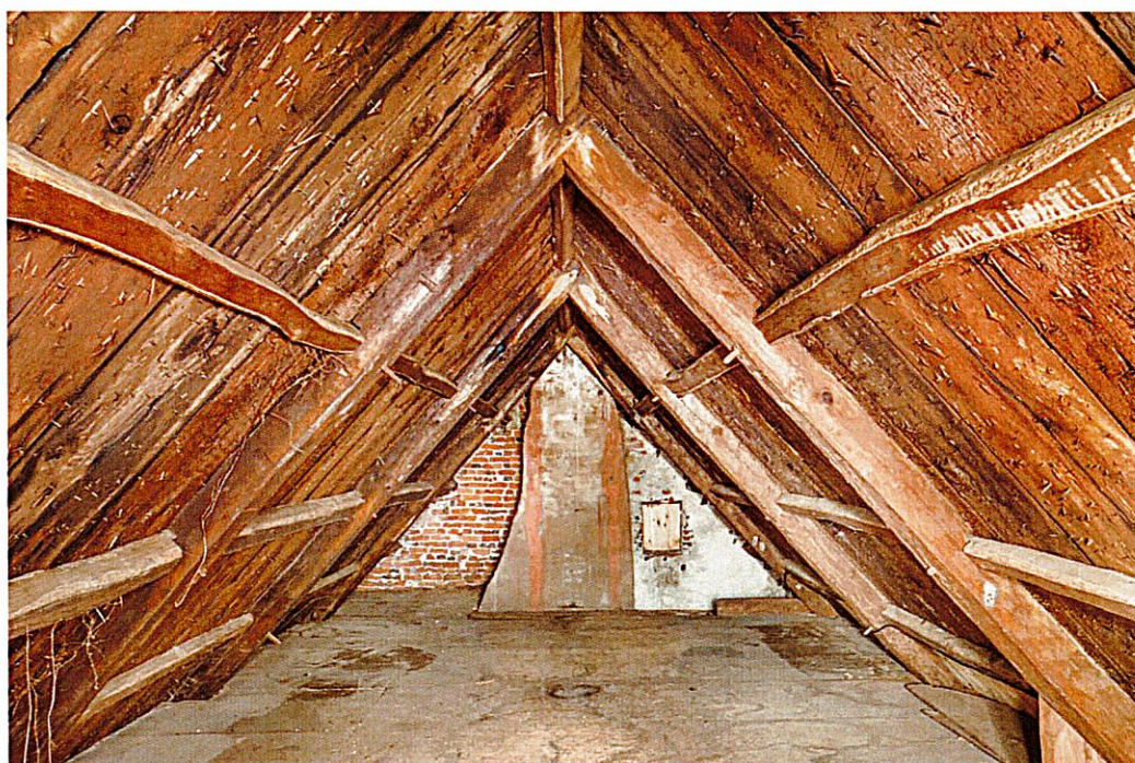
Exhibit B - MA: Haverhill, 790 East Broadway, PEASLEE GARRISON Rear Ell: Attic, looking north (RSID #502327)
