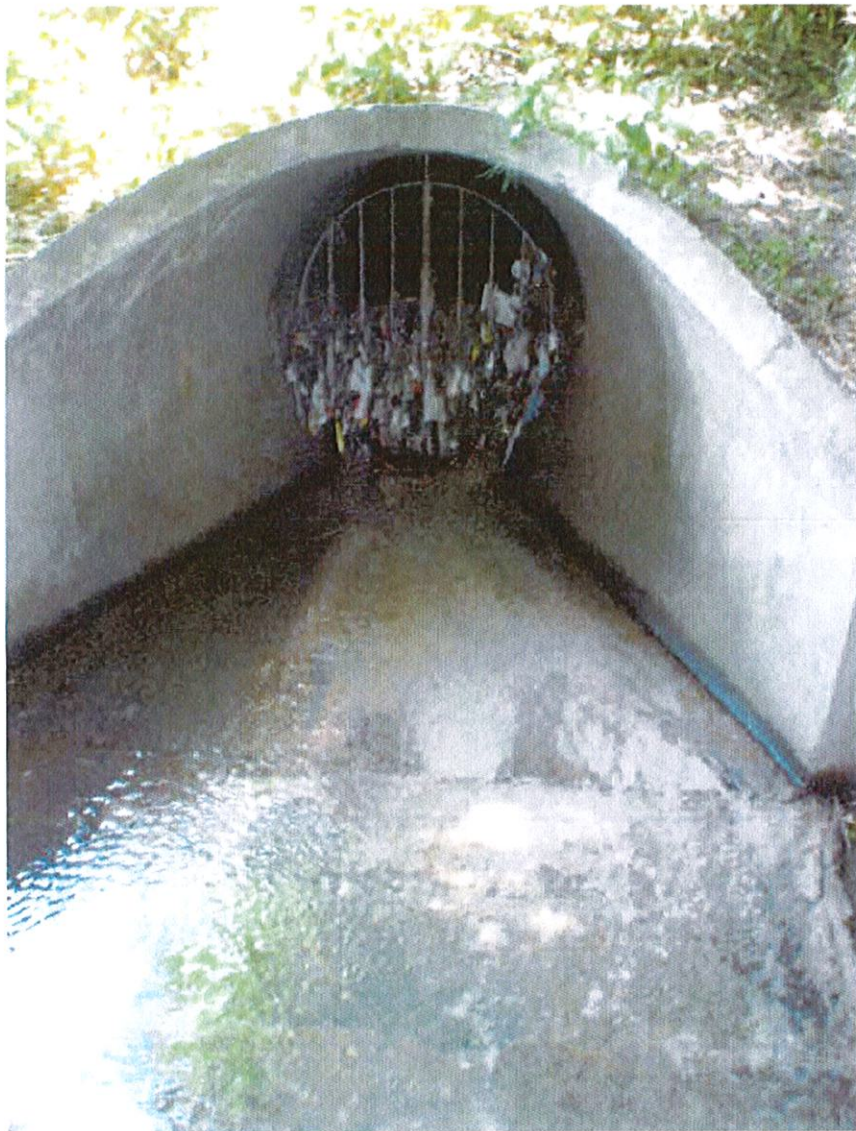
Note off-white filamentous bacterial growth
