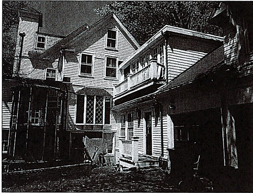
Facing the east side of the dwelling from the driveway.
