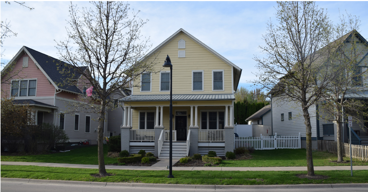
Two-story House with a gable roof and projecting porch.
