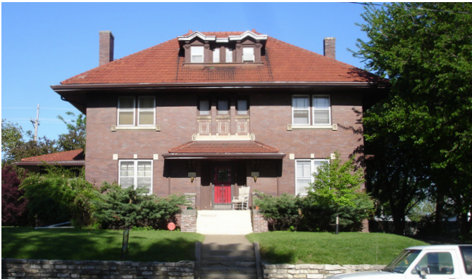
Two-story Duplex with a projecting porch.
