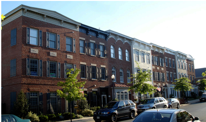
Three-story Townhouse Large with work activity on the ground floor.
