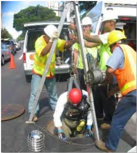
Photo 2-1. Confined Space Entry
