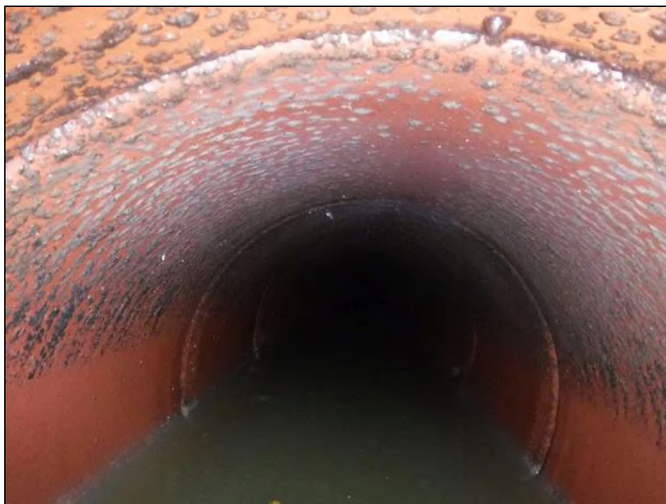
Monitored Northeast Influent Pipe
