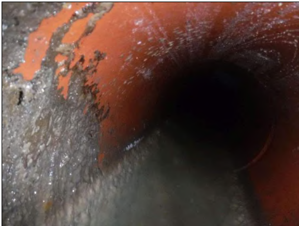
Northeast Influent Pipe
