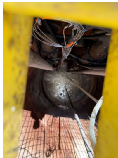
Wet Well, Piping and Valve Coating
