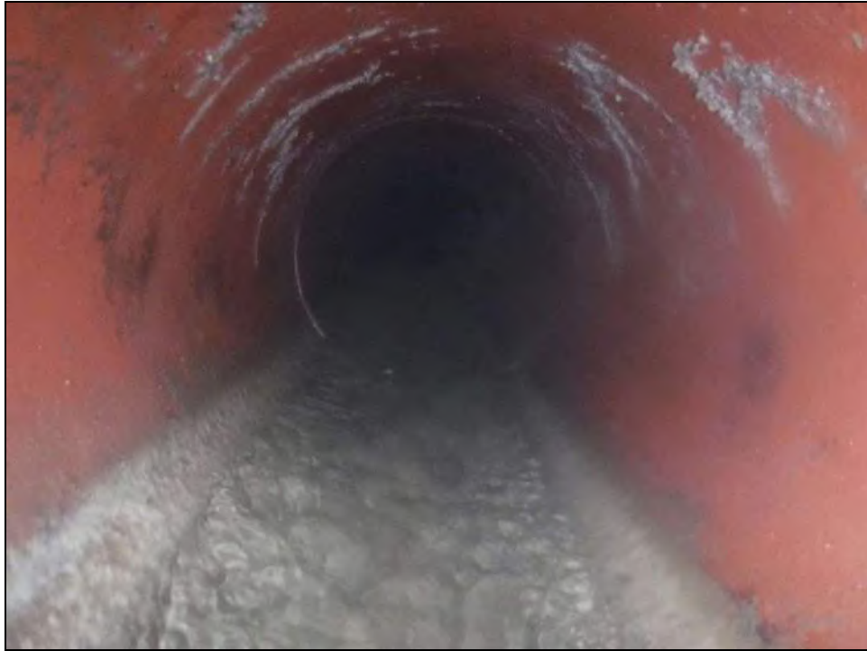
Northeast Influent Pipe
