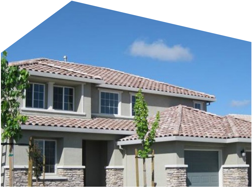
Tile roof on single family home.
