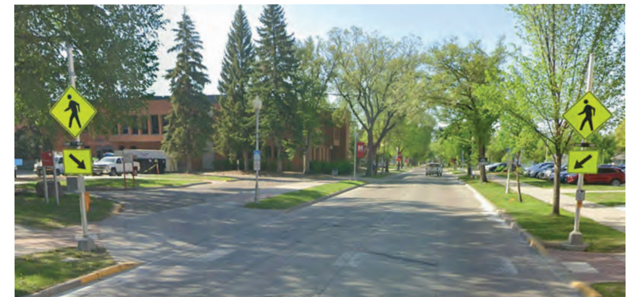
11th St Campus Pedestrian Crossing (Rectangular Rapid Flashing Beacon)
